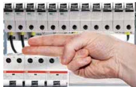
More working space between component rows.
