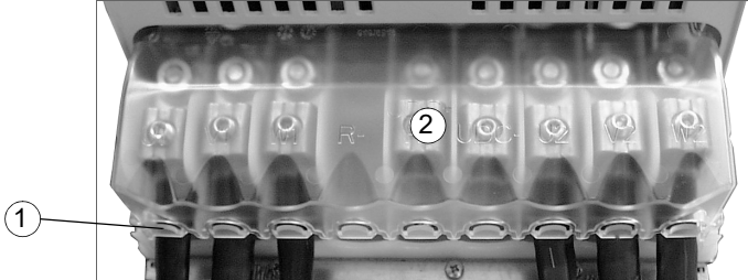
View of cable terminal installation
